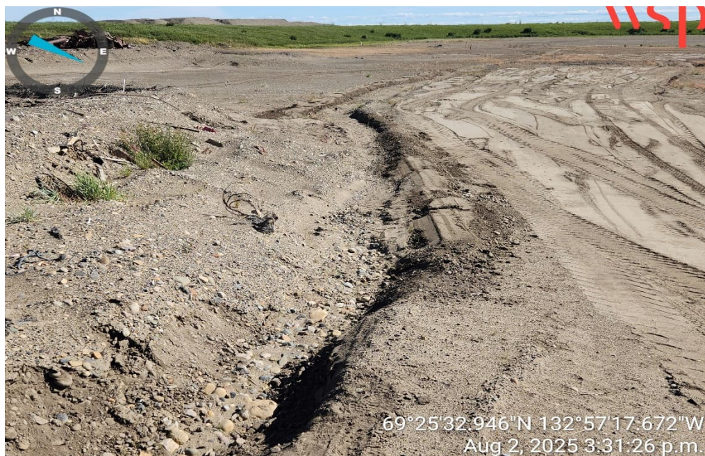
Photo 16 – Repaired swale along the west side of the South Landfill (2 August 2025).
