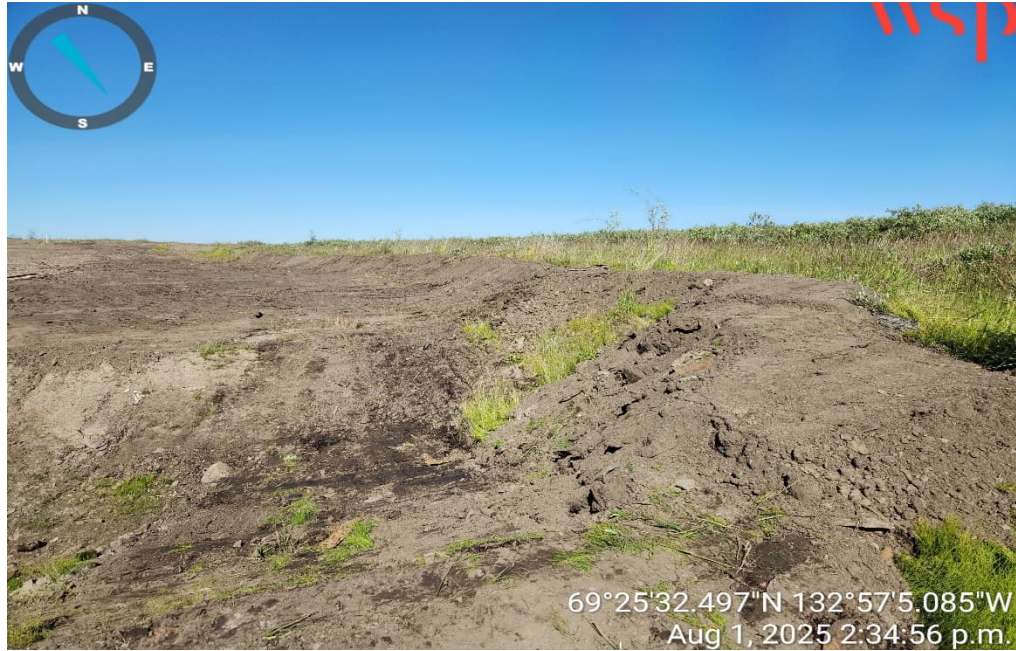
Photo 9 – Repaired berm along the east side of the South Landfill (1 August 2025).
