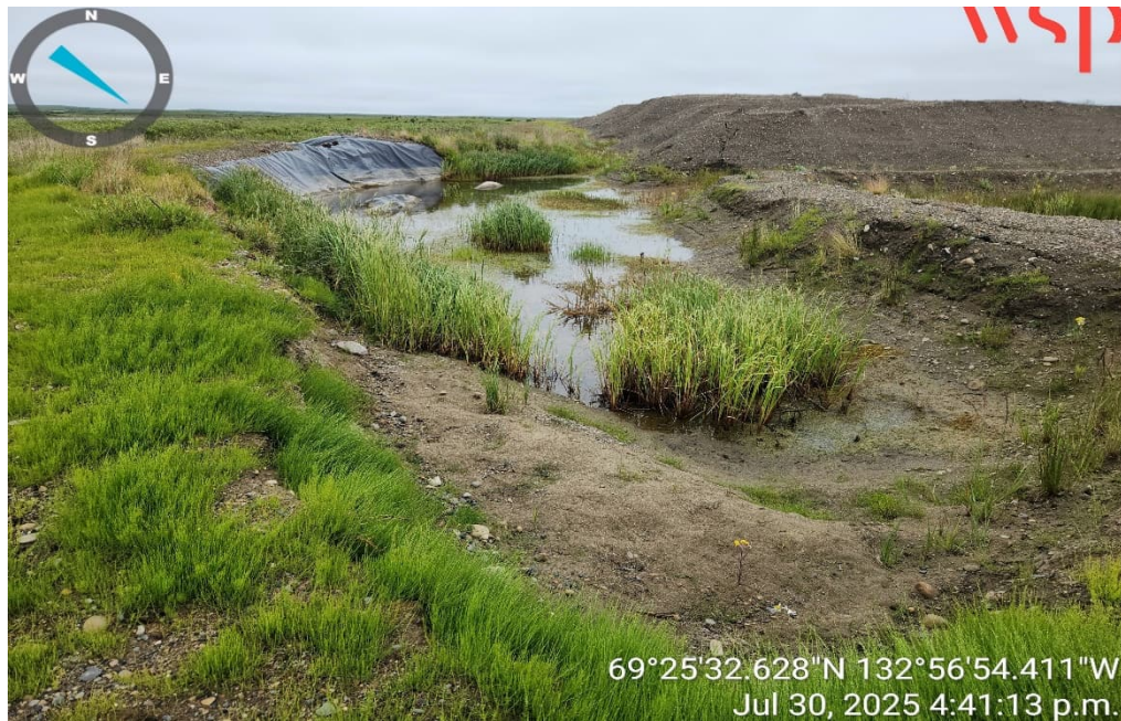
Photo 4 – Sump at ESSA 1 (30 July 2025).
