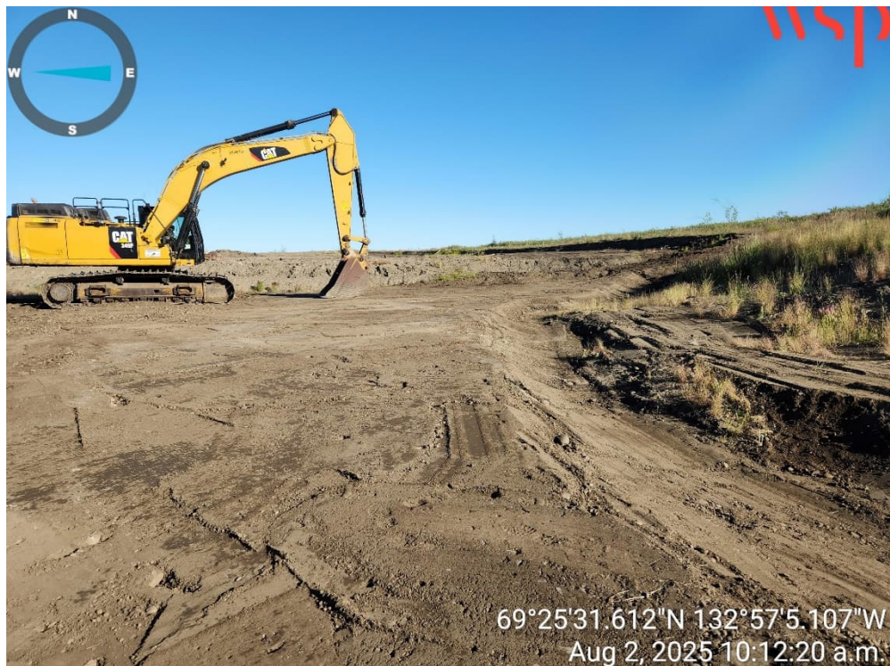
Photo 12 – CAT 349 excavator completing sloping away from the swale outside of the southeast corner of the South Landfill (2 August 2025).
