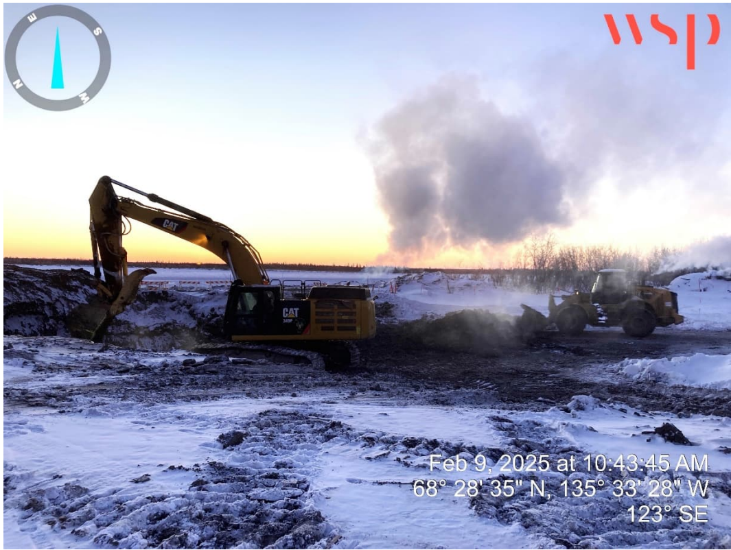
Photo 3 – Soil excavation activities (9 February 2025).
