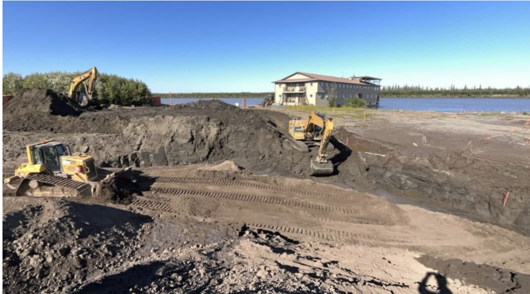
Photo 4 – Backfilling excavations with barge camp in the background (1 August 2025).
