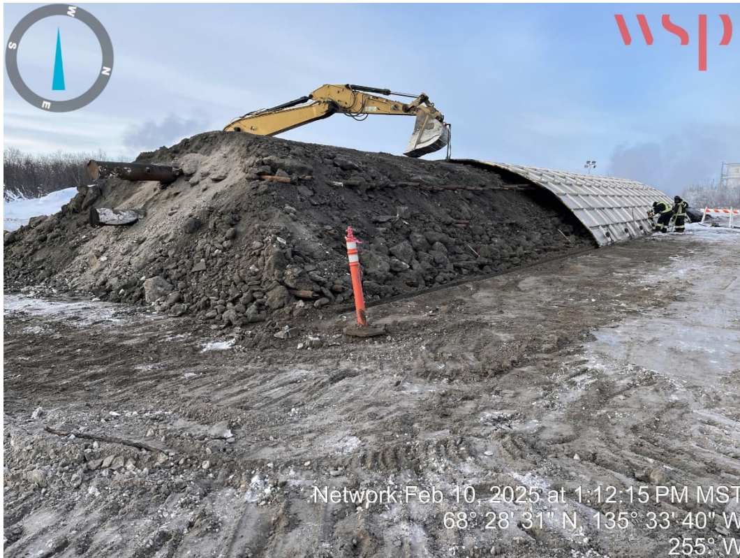
Photo 1 – Site remediation activities, soil treatment cell (10 February 2025).
