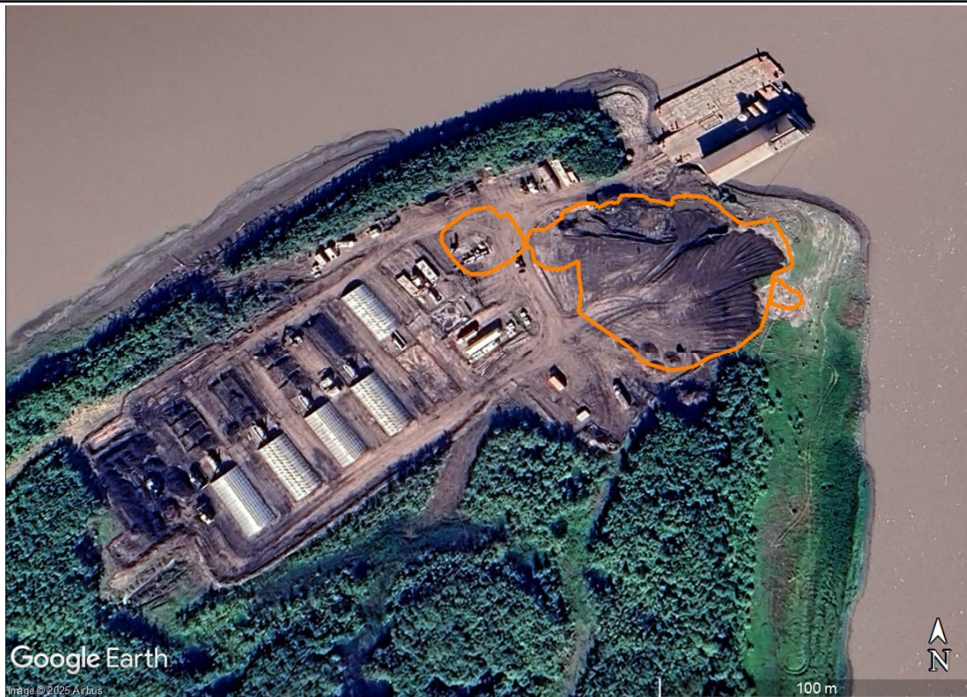
Photo 5 – Google Earth satellite image of West Channel from August 2025 with the final excavation limits as of October 2025 (orange outline).
