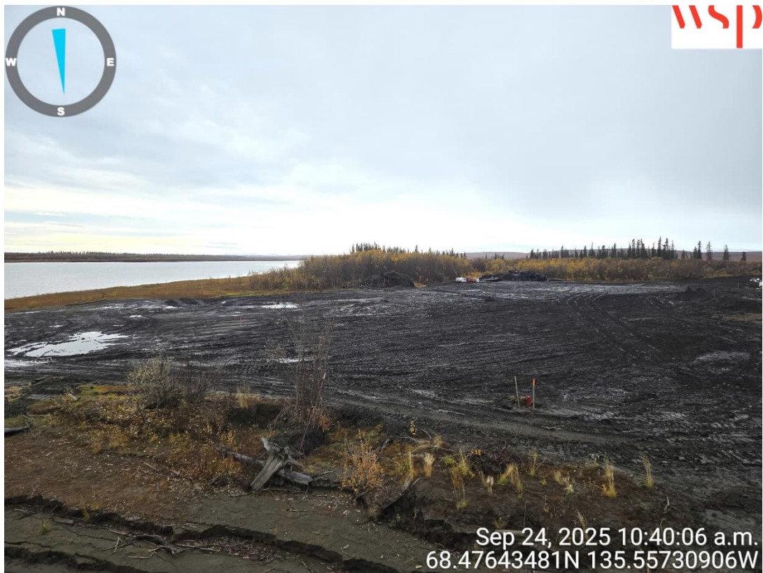
Photo 6 – Post-remediation, surface rough graded (24 September 2025).
