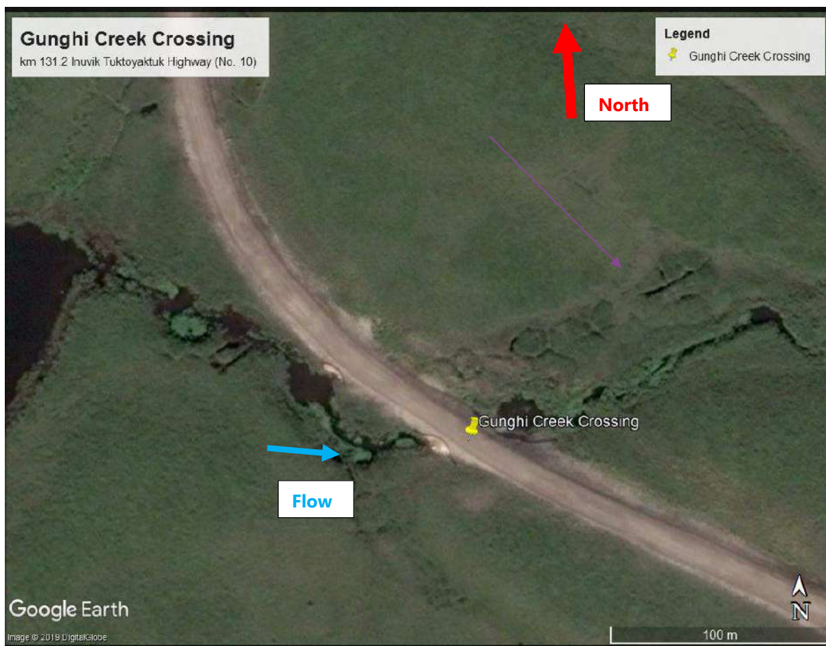
Figure 2-1 Gunghi Creek Crossing at km 131.2 ITH (No. 10)
