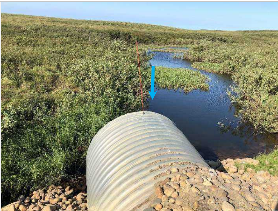
Looking west (upstream) Note Ponding and class 1M rock. Channel is not well defined. Photo taken July 25, 2019.
