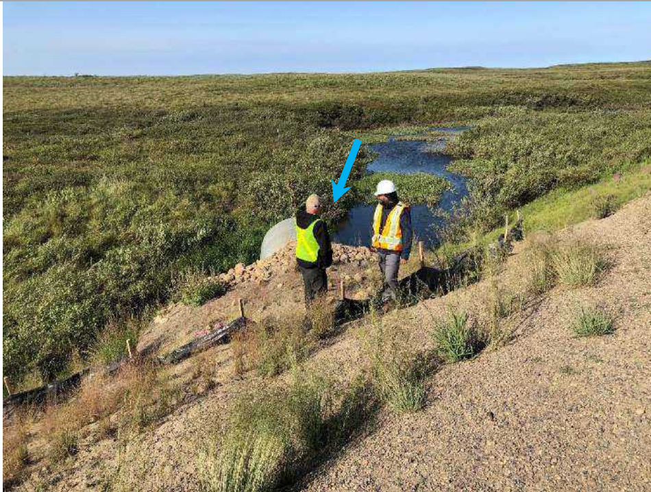
Looking west (upstream) Note Ponding and class 1M rock. Channel is not well defined. Photo taken July 25, 2019.
