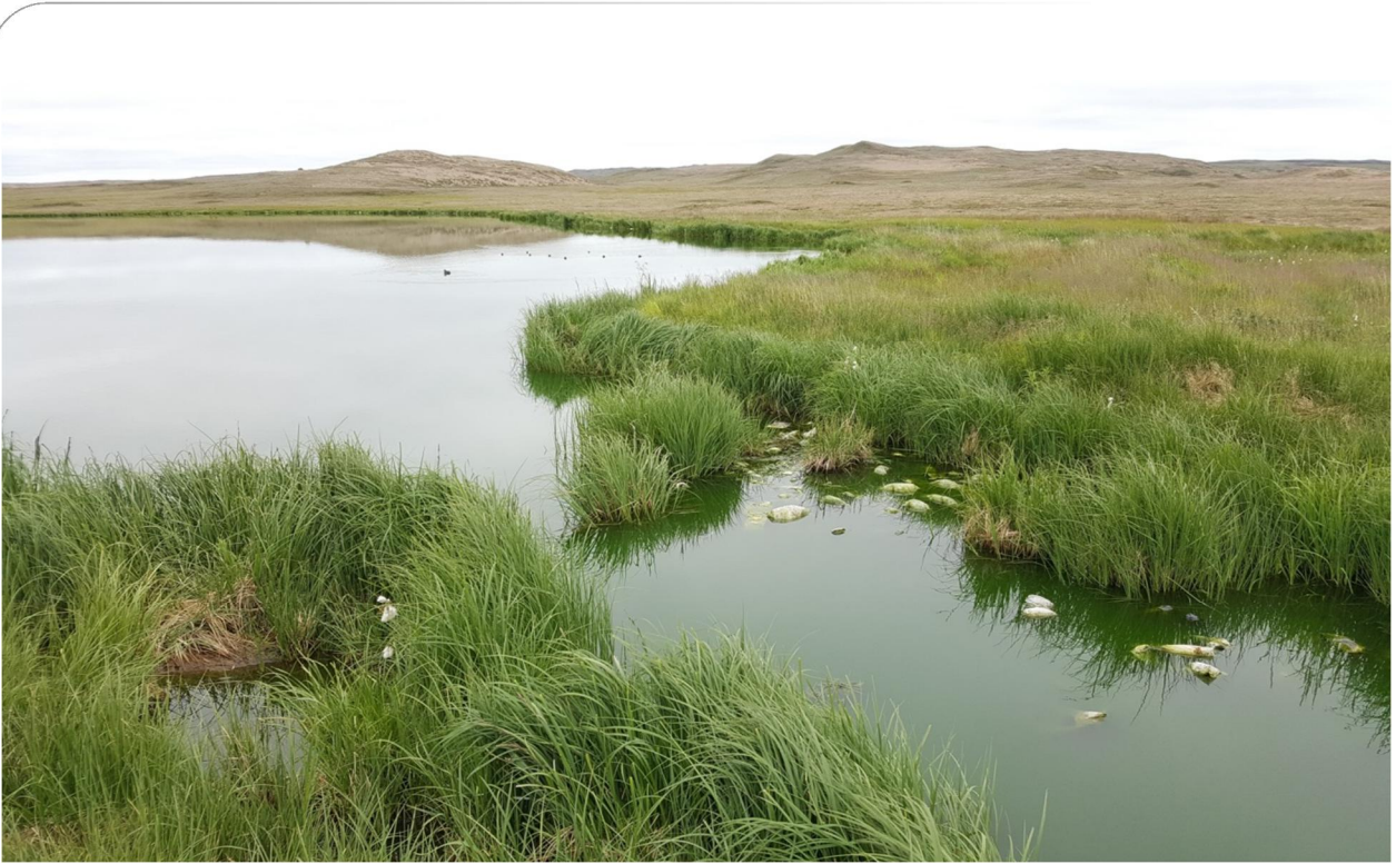
Figure 12: Sewage Lagoon Discharge to Wetland
