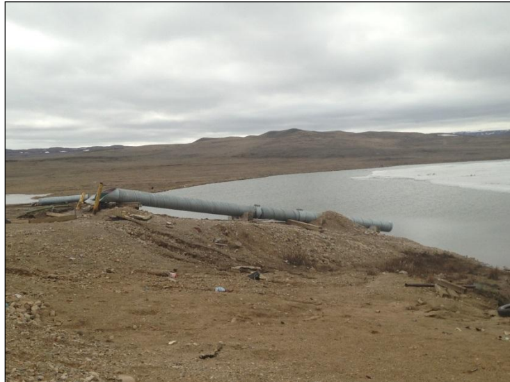
Figure 2: Paulatuk Discharge Chute (2015)
