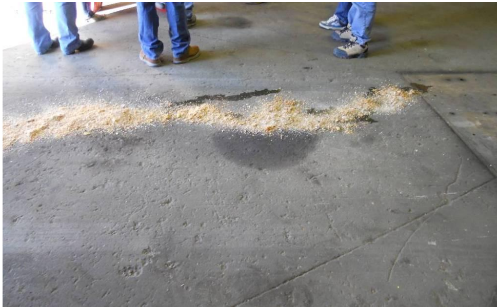
Figure 4: Absorbent Material Placed over Spilled Vehicle Fluids
