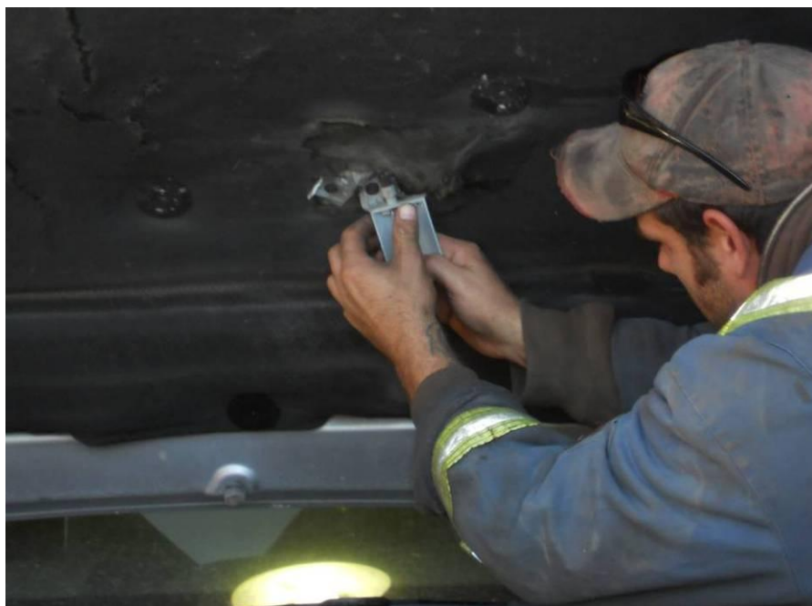
Figure 10: Example of Removing Light Assembly Containing a Mercury Switch
